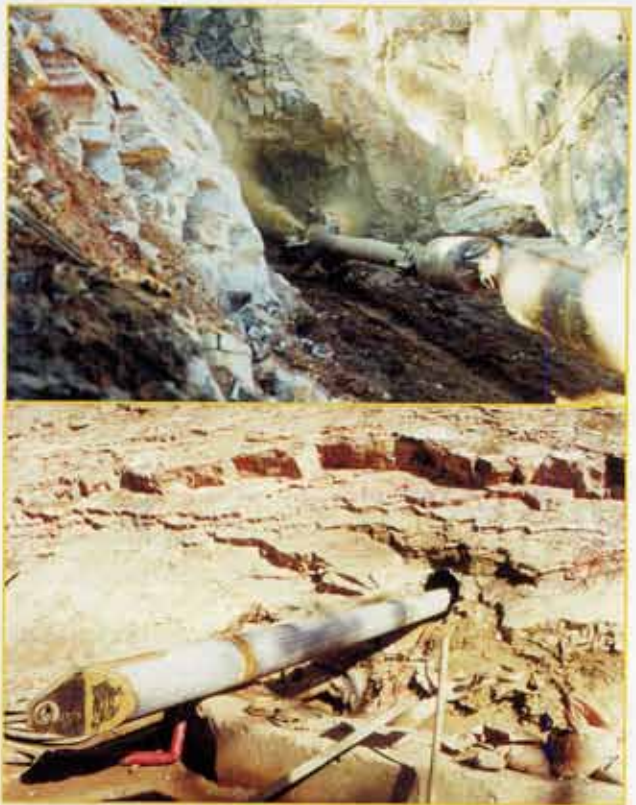
Figures 6 and 7. Pipe pulling operations.
