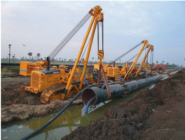
Figure 2. 48 in. pipe tail during pulling.
