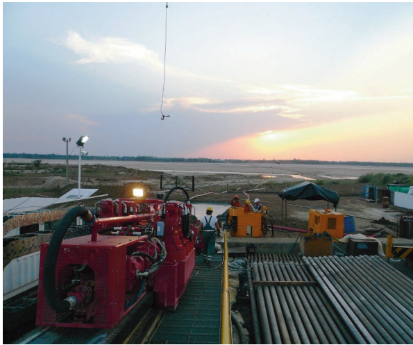
Figure 3. 400 t rig set up on the Vashishta bank.
