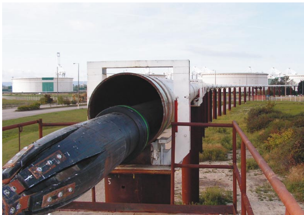
Figure 5. Pulling the buoyancy control system inside the 34 in. pipe-string.
