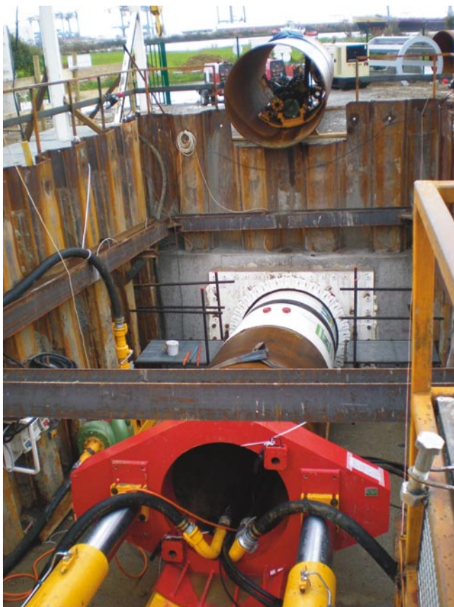
Figure 4. Installing one of the 66 in. entry shafts.
