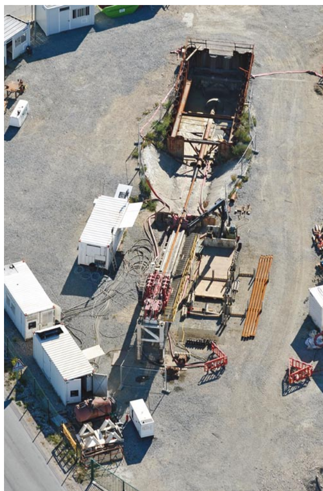
Figure 6. Spread HK 400 and entry shaft at north side of the crossing.
